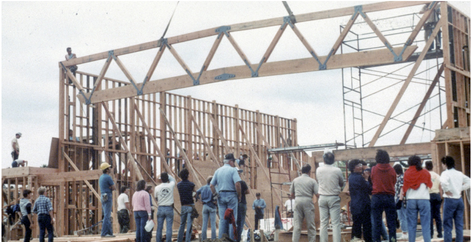
The first truss of the Activity Center hoisted up (first building, 1986)
